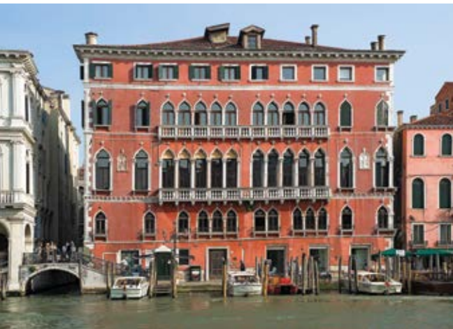
Palazzo Bembo, where the UB exhibit is housed.
